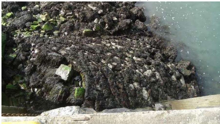
View looking down from quayside at the embrasure feature built in front of the stone quay at its southern end, to act as an armoured protection.
