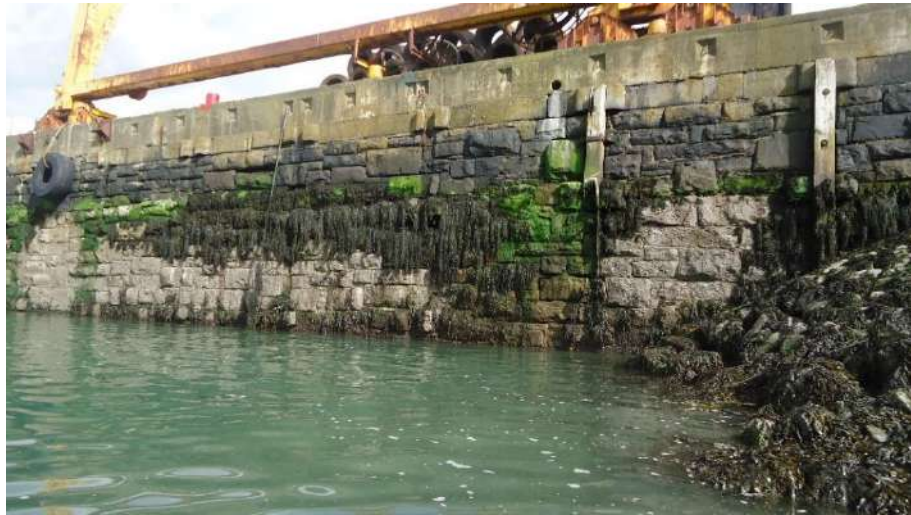
View along the façade of the stone-built quay in 2017, showing the cut stone blocks and the projecting jamb stones in the upper level spaced at regular intervals to secure the vertically-set timbers used as fenders. The uppermost layer of concrete was a later addition to support that quayside cranes in use.
